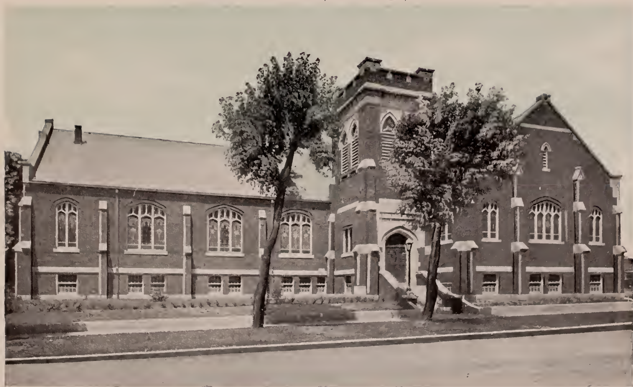
FIRST PRESBYTERIAN CHURCH, MARSHFIELD, WIS.—26
